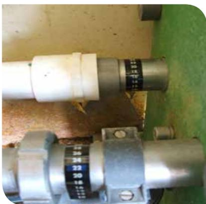
**Figure 1:** Is your plate cooler taking enough heat from the milk? At 6°C difference this system needs checking.
